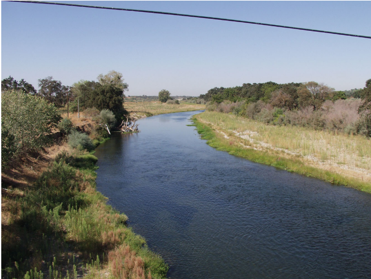
Figure 61. View of completed reconstruction of the 7/11 Reach looking downstream from the Roberts Ferry Bridge (RM 40.3).
