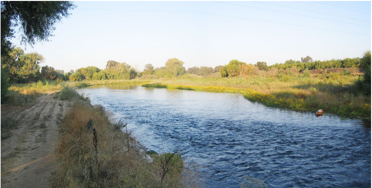
Figure 70. Construction (summer 2001 and as-built (summer 2003) ground photographs of SRP 9, looking downstream from west side of Geer Road Bridge.
